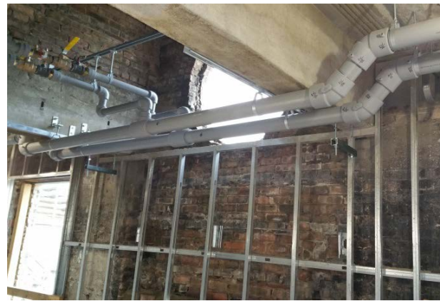
Photo 2: PP-RCT Pipe installation for an elderly home
